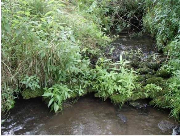
Shale weir related to a forebay
